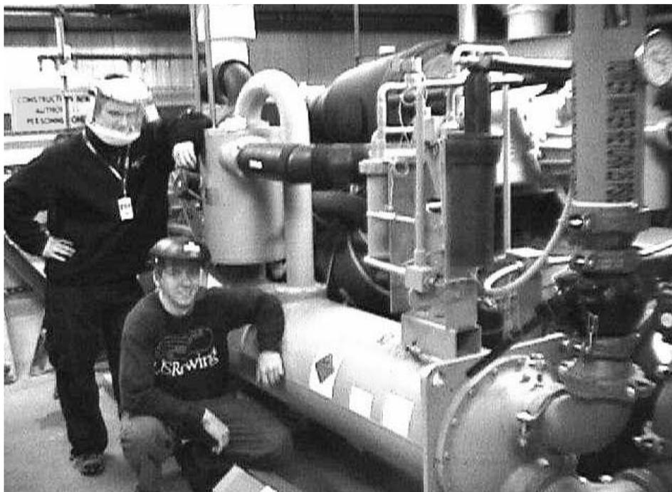
Creighton physics majors, **Peter Dudley** (left) and **David Lynch**, are shown inspecting the cooling system for the magnet coils of the STAR Detector at Brookhaven. The main coils carry 4500 amps at 575 volts!
